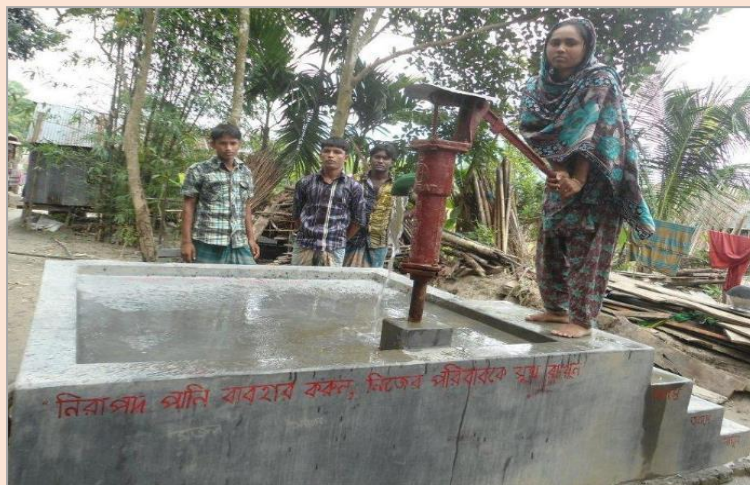
Fig. 6: Example of improvements to rural water sources identified and implemented through the WSP process; a tube well raised above the flood level.
