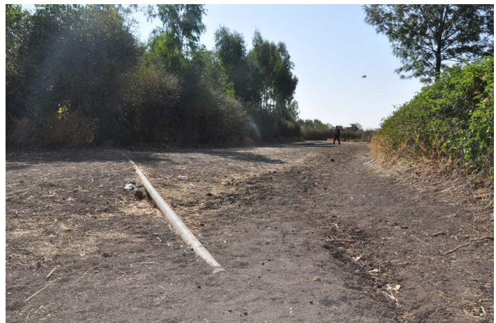
Water pipes that are exposed in the open is common in many places during the assessment
