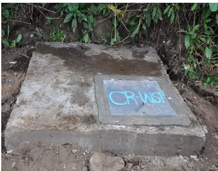
Manholes covered with metal sheet that prevent contamination and eases maintenance
