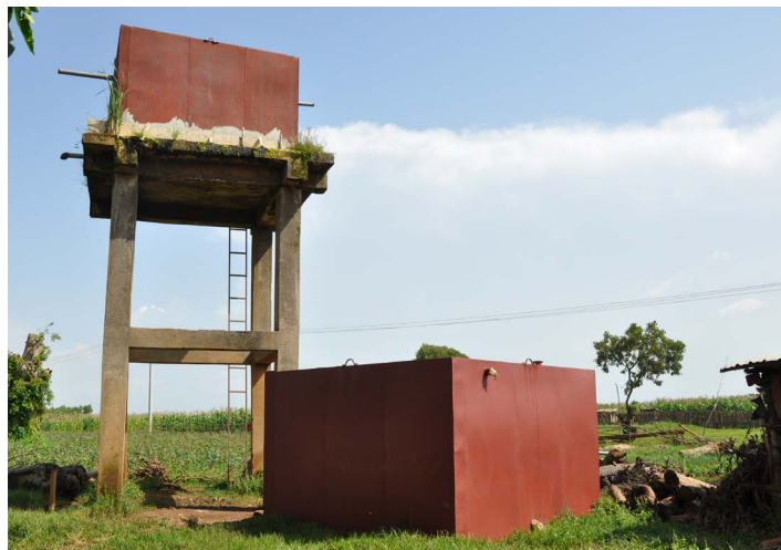
This water tanker was leaking and has been rusted for many years in Lalibela Kebele of Amhara region. They have recently ordered a new one and ready to substitute it.
