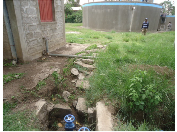
Field visit on CRWSP, open inlet manhole in one of the reservoir at Butajira town, photo Osman WHO, 13 June 15
