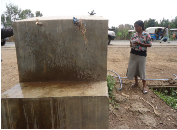
Field visit on CRWSP, public water point with no fence, open manhole with full of dirt and damaged faucet, Butajira town, photo Osman WHO, 13 June 2015
