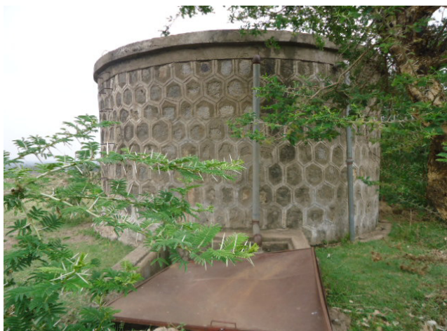
Field visit on CRWSP, reservoir with no fence and damaged manhole, Ellie kebele, photo Osman WHO, 11 June 2015
