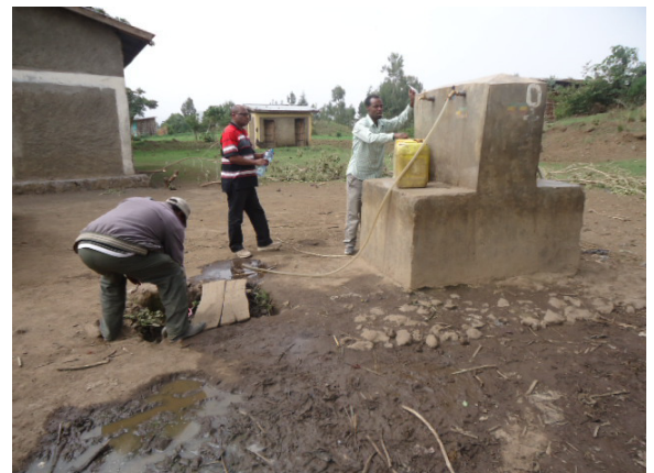
Field visit on CRWSP, public water point with no fence and open manhole around a health post, Butajira town, photo Osman WHO, 13 June 2015
