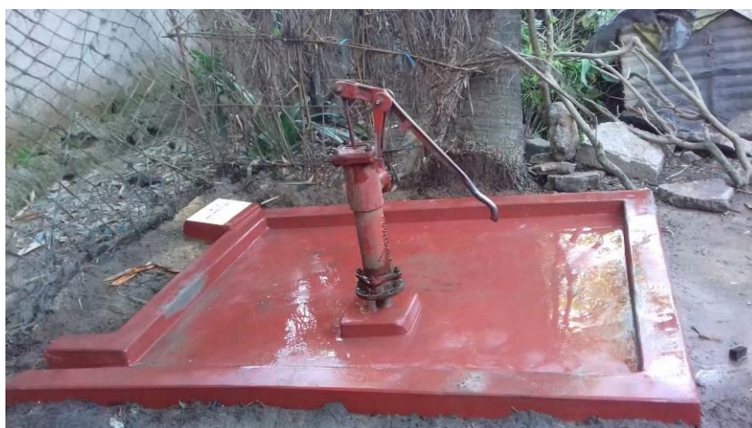
Demonstration of renovation of TW platform
