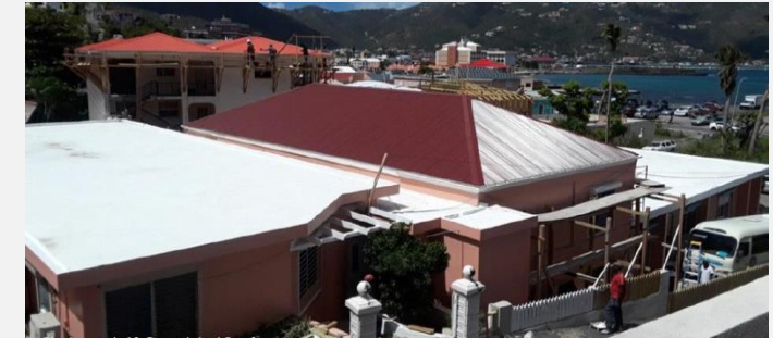
Strengthened roof with cool coating
