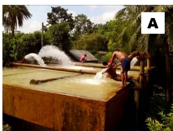
Fig. 6.3: Photograph of treatment plant A: aeration chamber, B: chlorine dosing, C: Overhead tank
