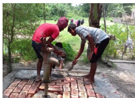
Renovation of Tube well Platform
