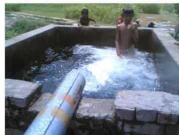
Deep Tube Well with Unprotected reservoir
