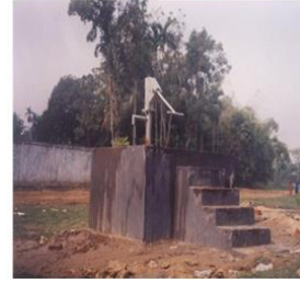
Raised Tube well in flood Area
