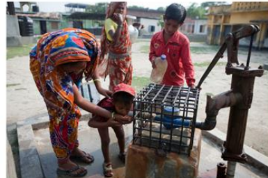
Boreholw with Protected Chlorinator Ionizer
