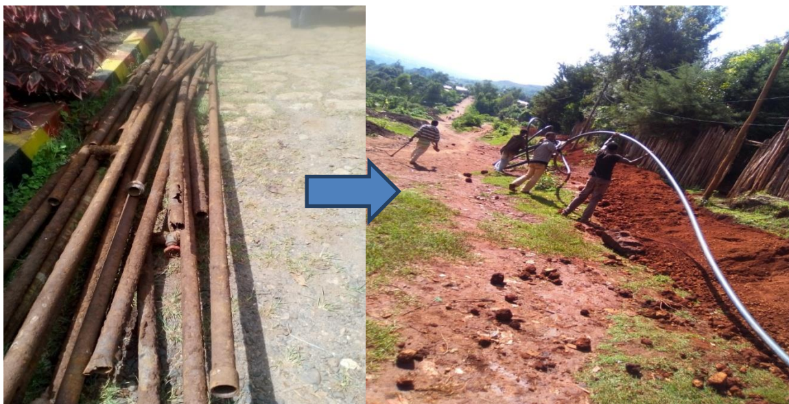
Photo 4 Damaged galvanized pipes replaced by HDPE, more than 1.2 km, Wolaytasodo
