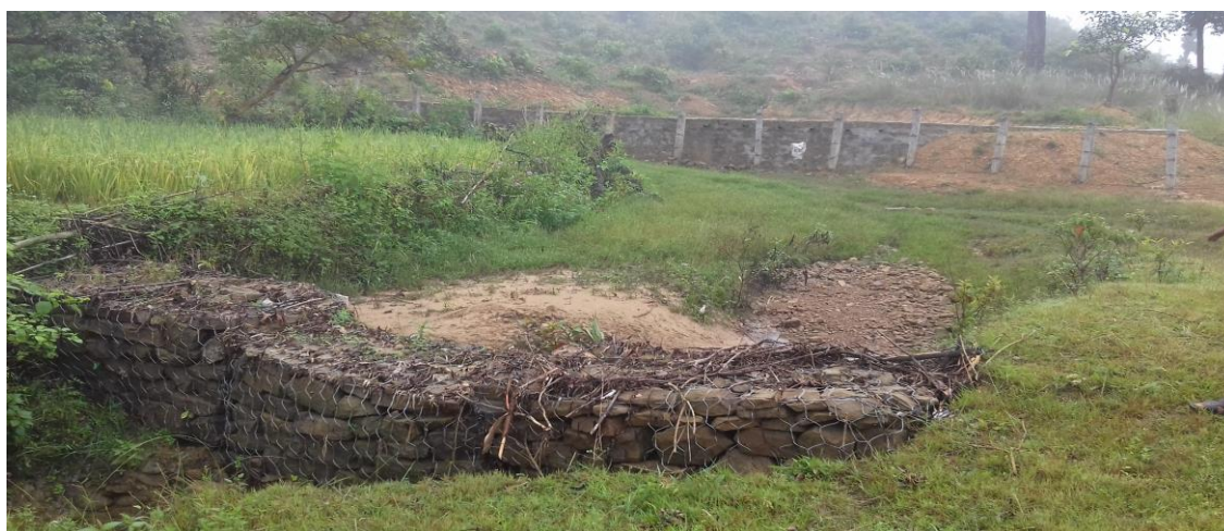
Fig. 18: Gully Treatment
