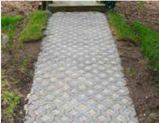
Installed permeable pavers 17
