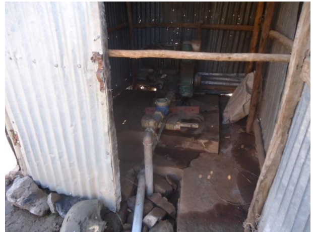
A deep well water source with cracked/damaged well head Fatsi town, photo Osman WHO, 27 Dec 2015
