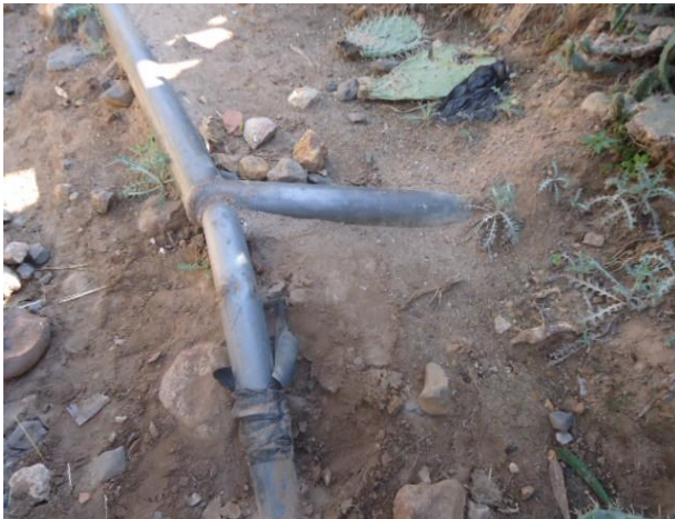
Damaged pipeline and covered with plastic: CR-WSP training, Adigrat town photo Osman WHO, 21 Dec 2015
