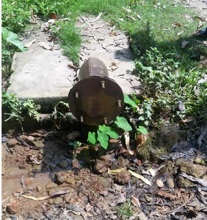
Figure 6: Wash out chamber in Pourashava water supply system
