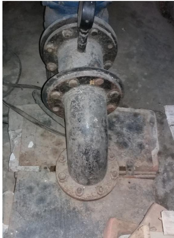
Figure 7: Sanitary seal for production tube well in pump house
