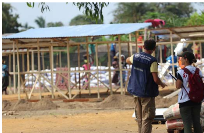
Technical discussion between WHO and MSF on the construction of the new Ebola treatment centre in Bulape, Democratic Republic of the Congo – September 2025. © WHO
