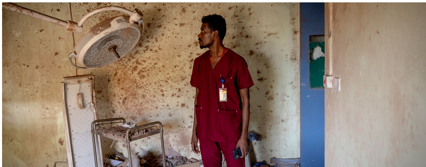
A health worker stands in a destroyed room at Aalia Specialist Hospital in Omdurman, Sudan on 21 April 2024. Credit: Ivor Prickett/The New York Times
