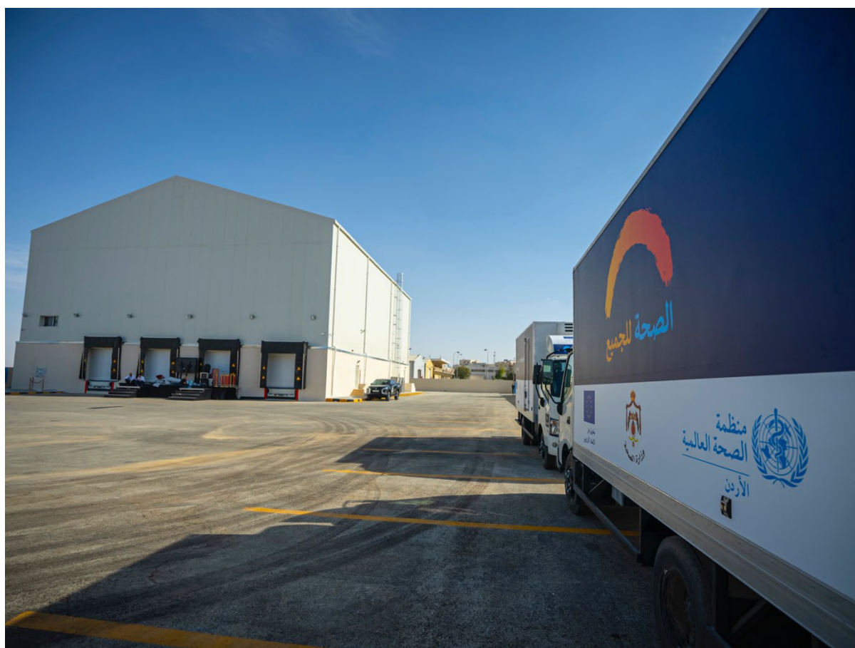
An ultra-modern warehouse in Jordan, with transportation supported by WHO through the EU Trust Fund. ©WHO
