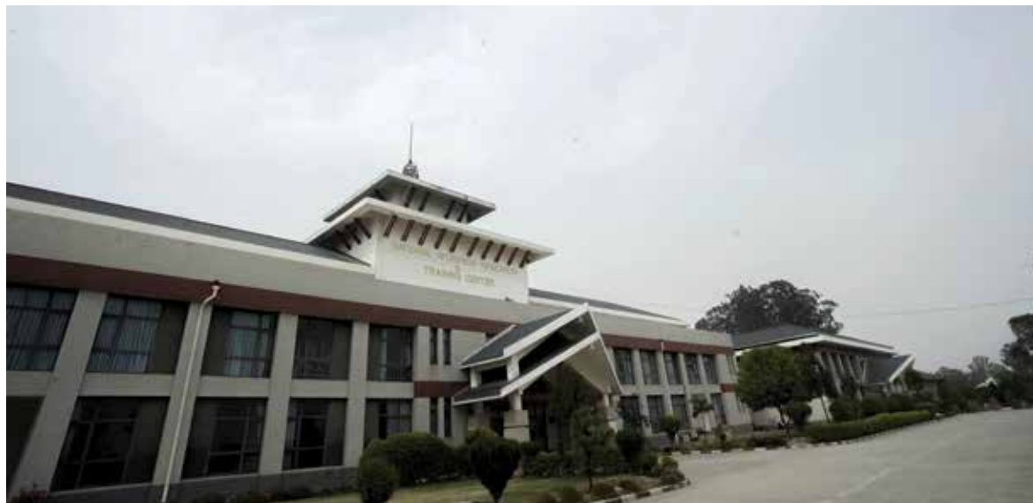
◀ A scene outside of the National Ayurveda Research & Training Centre, Kirtipur, which functioned as an isolation facility for patients diagnosed with COVID-19.
