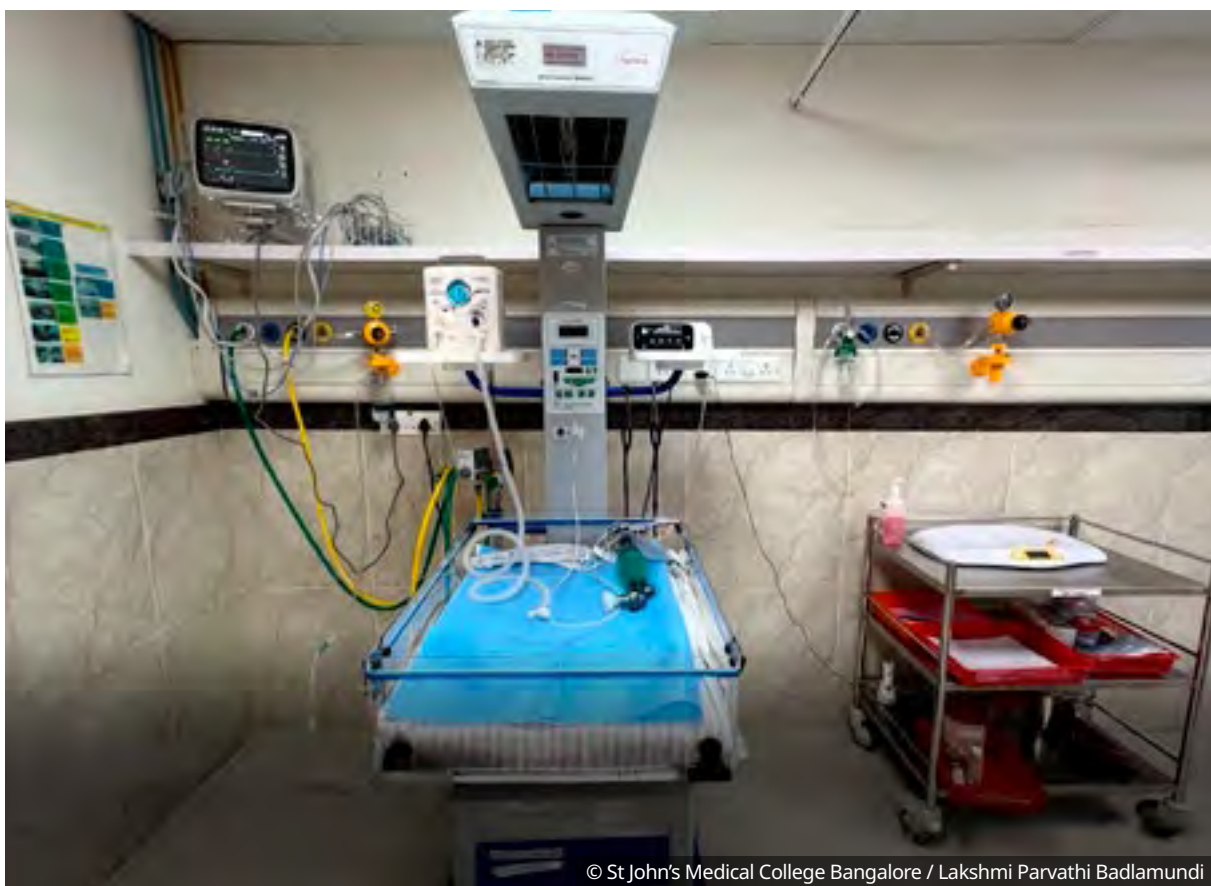
Setup of a newborn resuscitation area in a level 2 health facility
