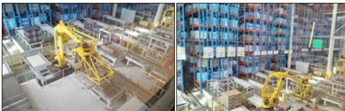
Figure 18. Warehousing palletizer and automated storage and retrieval system
