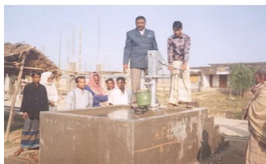
Fig11: Photograph of raised platform of tube well
