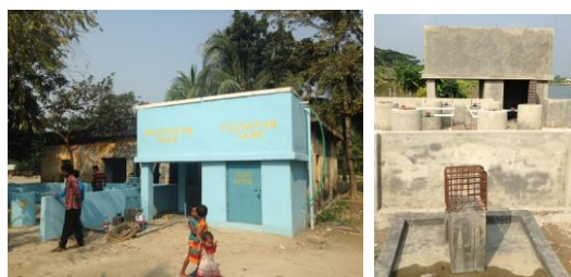
Fig. 12: Photograph of aquifer recharge system
