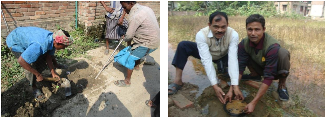
Figure 4.8: Cleaning of old sluice valve chambers (left) and repair wash out pipes (right)
