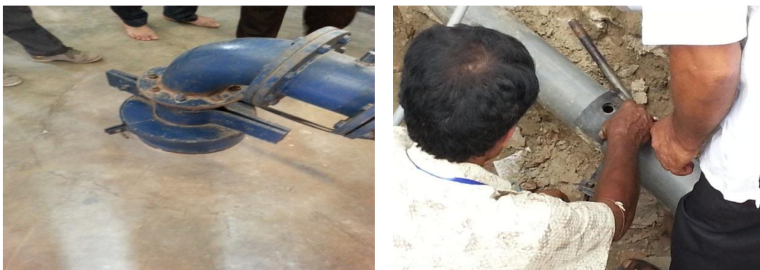
Figure 4.9: Pump house and sanitary seal after cleaning/repairing (left) and use of pipe driller during providing house connection (right)
