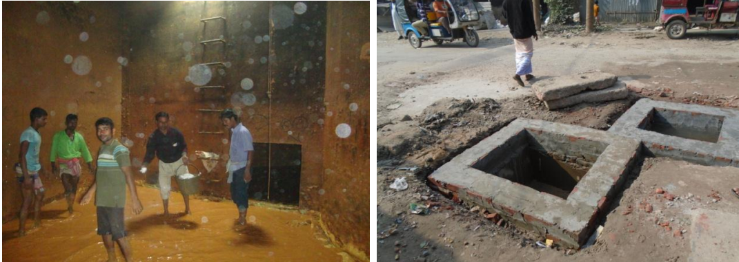
Figure 4.7: PWSS staff cleaning overhead tank (left) and newly constructed sluice valve chamber (right)
