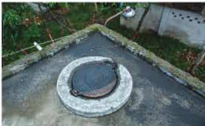
Manhole is slightly raised than the top surface of the reservoir and it is covered firmly with a lid
