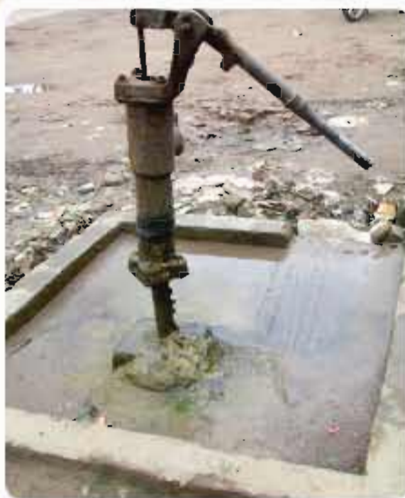
Tubewell platform is unclean and/or water stagnates on it
