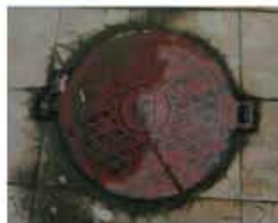
Opening of manhole is at the same level of the top surface of the reservoir
