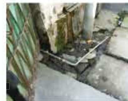
Weak joints in pipeline at drain crossing
