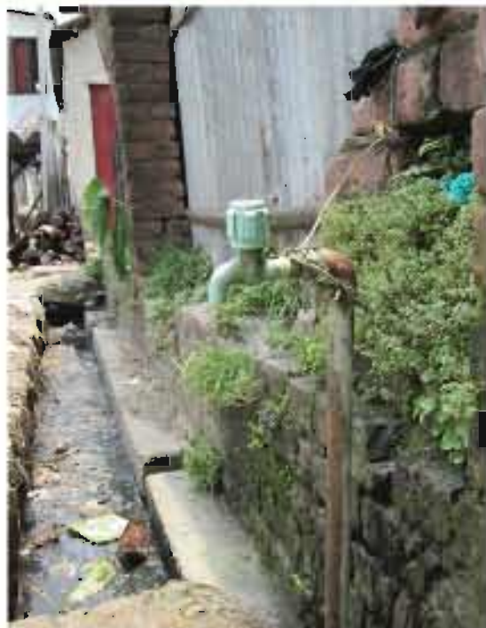
Tap-stand is placed adjacent to waste drain; platform of the tap-stand is broken or missing; water stagnates at the base of the stand
