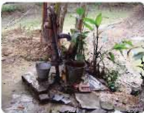
Tubewell platform is damaged or missing
