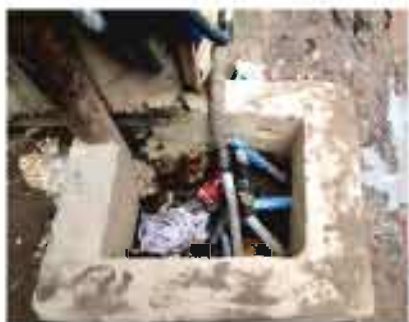
Water connections is not made properly with standard material
