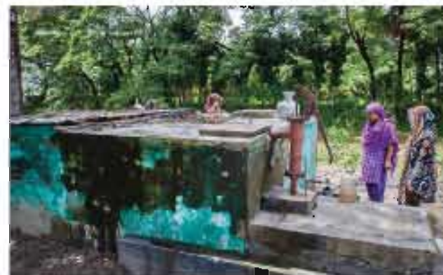
Platform of PSF is broken or unclean or lichen has grown on the surface of filter chamber
