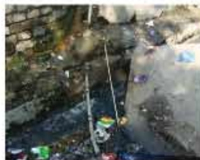
Pipes are not well protected while crossing canal/drain
