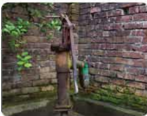
Dirty plastic bottle or part of it is attached with the spout of tubewell
