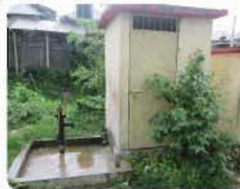
Latrine exists within 30 feet of the tubewell
