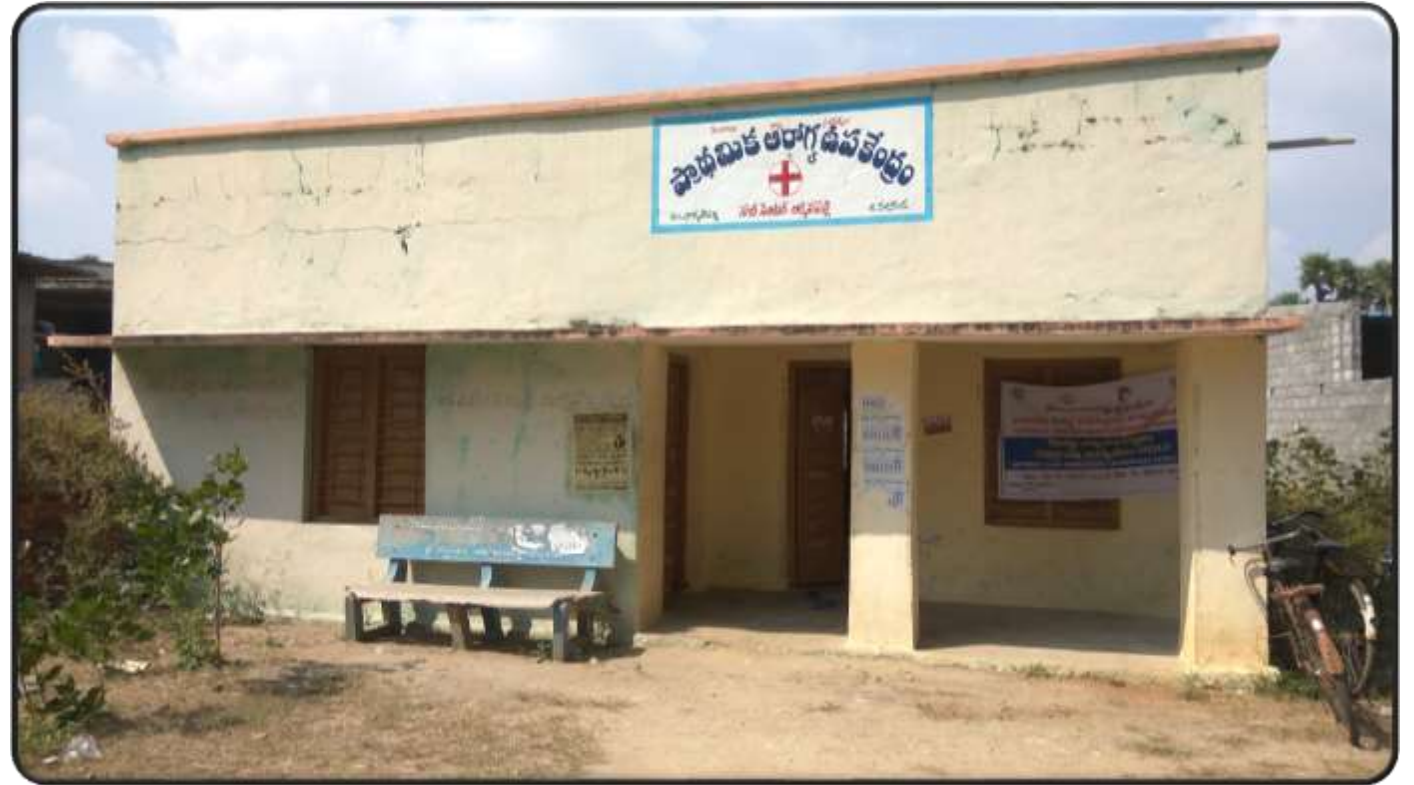
A Primary Health Center in South India
