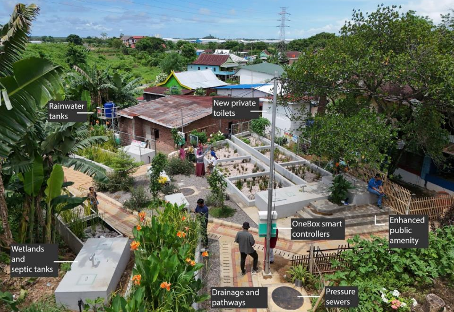
View of the tailored RISE water-sensitive upgrading intervention in an informal community. Makassar, Indonesia: 2024. © RISE.
