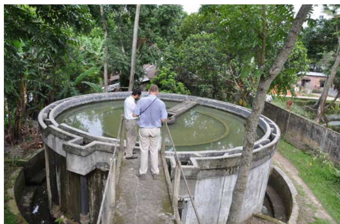
Treatment works inspection at Chandpur Paurashva treatment plant, Bangladesh. © WHO/Payden.
